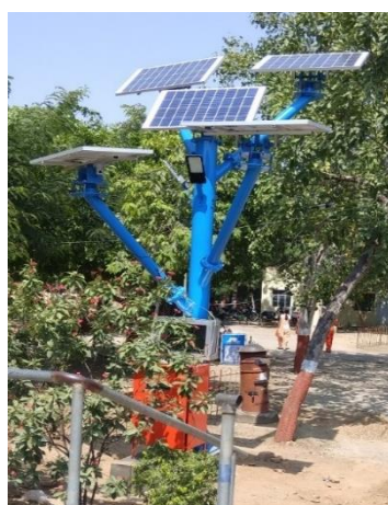
Figure 1. 500 W solar tree installed at CSIR-CEERI, Pilani
