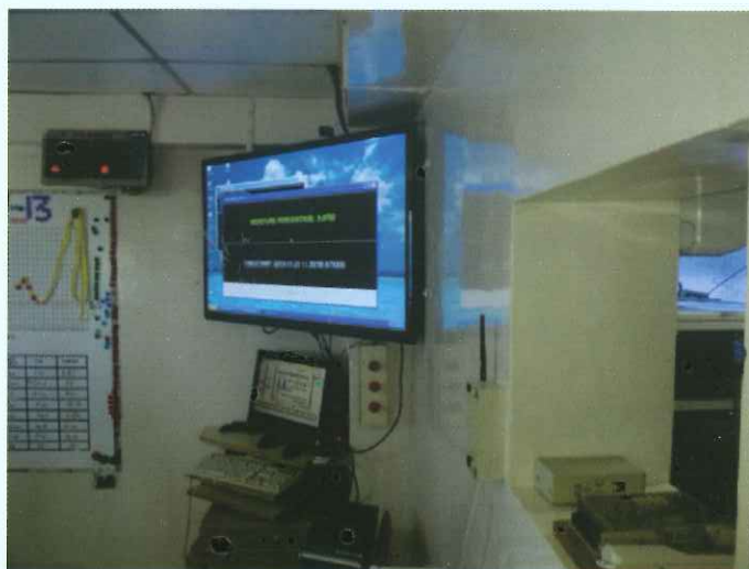
Figure 5: Display of moisture values in the control room relayed wirelessly by the moisture sensor
